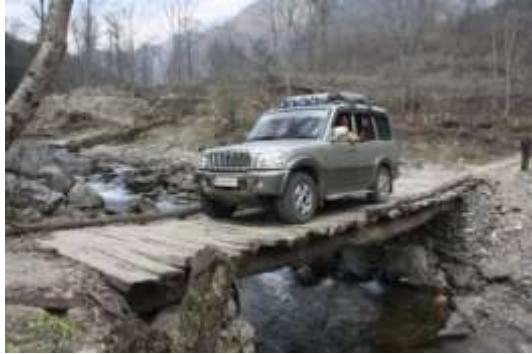
Dodgy bridge on the road to Eaglenest
